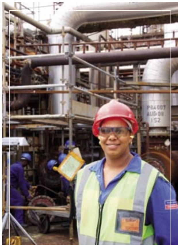
Raazia Harris, Safety Watcher, with contractors opening a heat exchanger prior to decoking.
