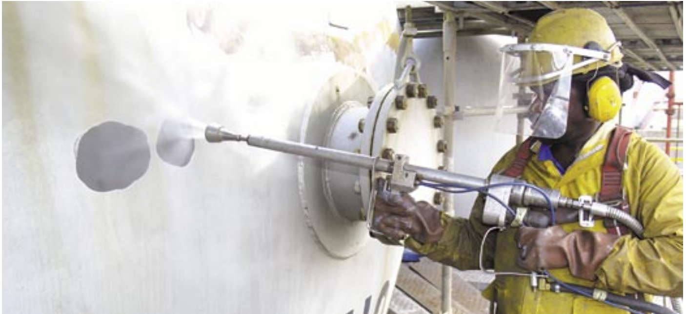
Alson Dlangalala, a UHP blaster at Kaefer Thermal, UHP water-jets the surface of a vessel prior to the application of a coating.
